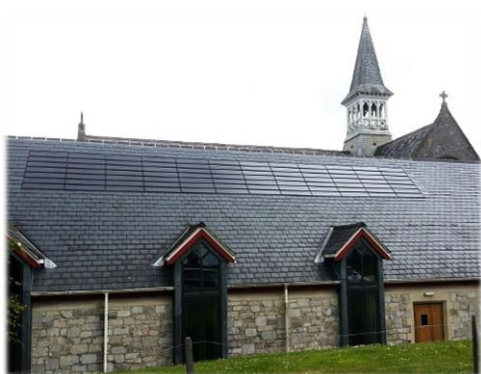
Image of Solar PV slates on a grade I listed church in Devon
