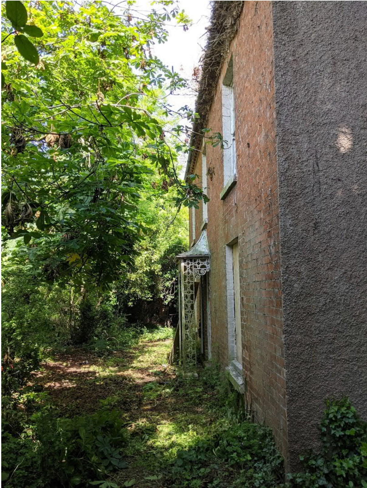
7.20. The brickwork front is in fair condition. Some plant growth is evident which will be causing damage. There is extensive ivy growth visible at the eaves which has damaged the gutters and roof.
