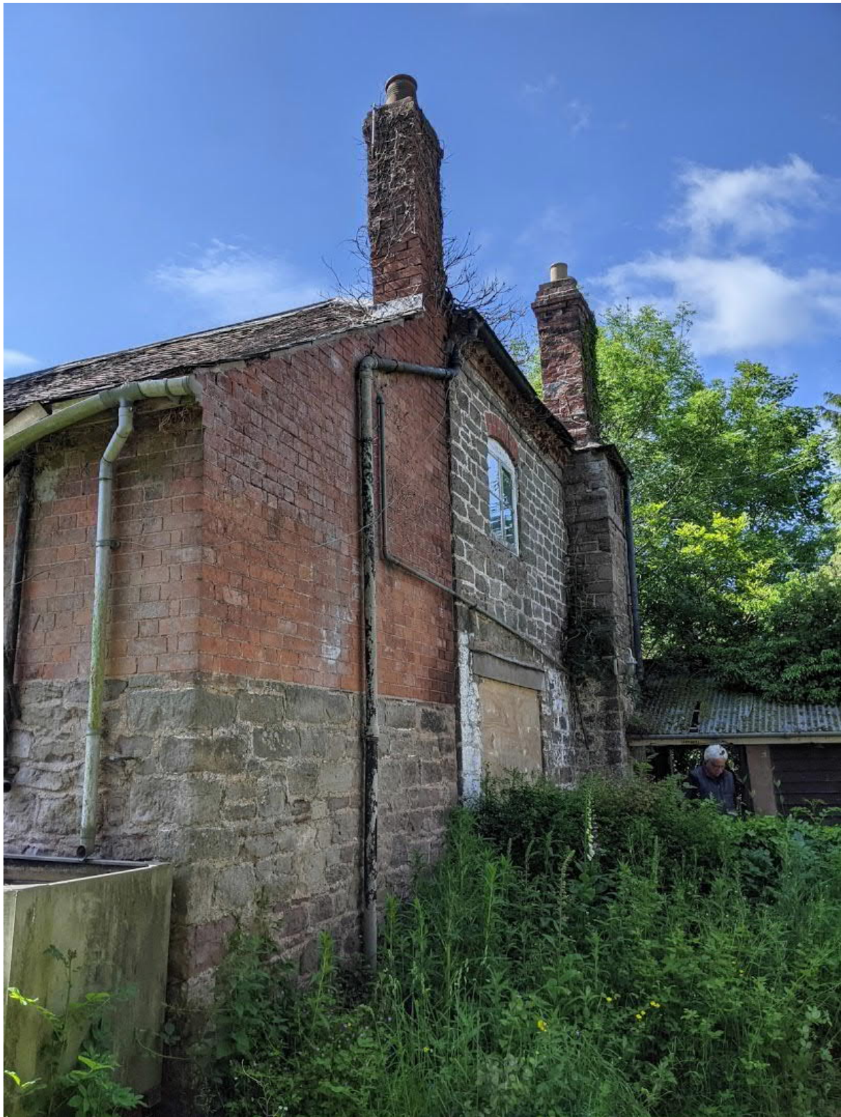
7.23. The west elevation has the most varied stone condition. It appears that the stonework and masonry is of varying age suggesting that the structure has been historically altered.
