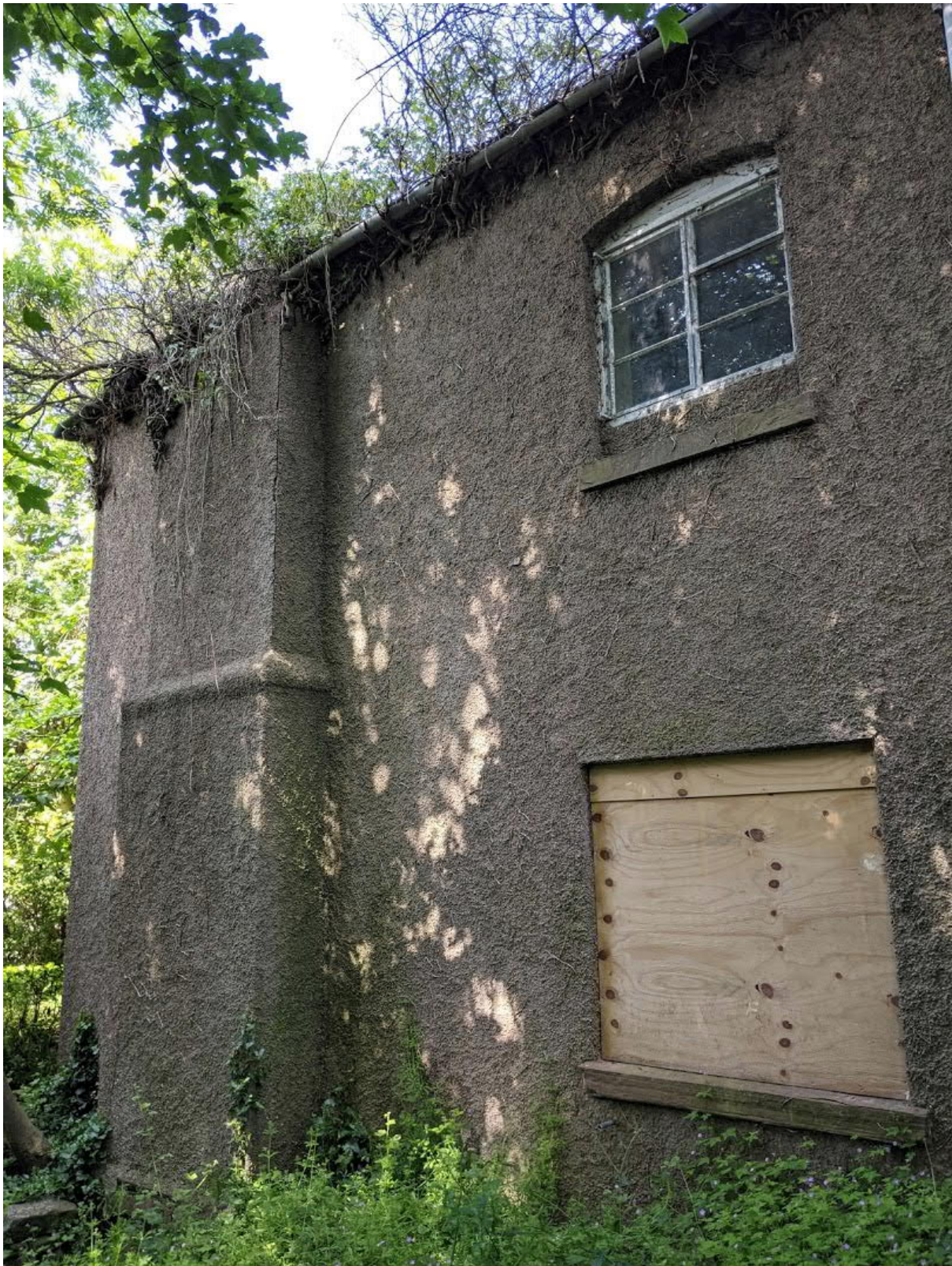
7.17. The Eastern elevation has been rendered. The render cover seems relatively good with only a few visible cracks. There is extensive ivy growth visible at the eaves which has damaged the gutters and roof.
