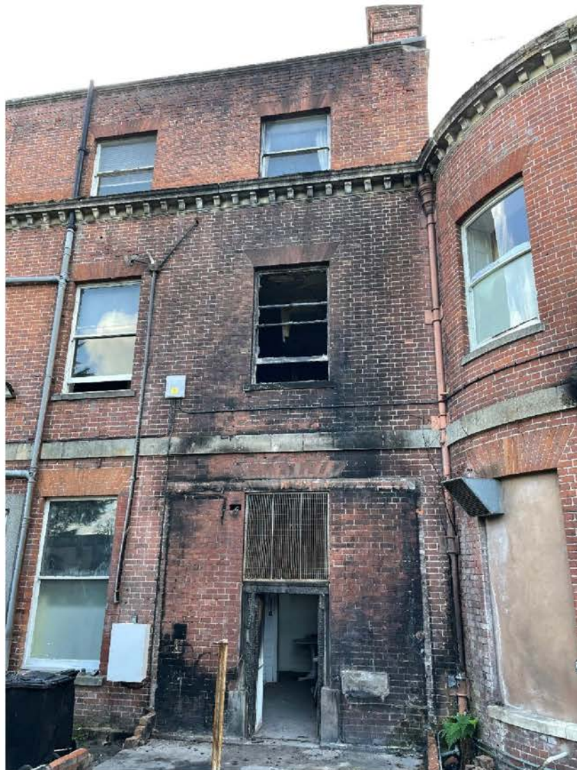
Figure 6 – Close up of damaged area to rear elevation and previous location of conservatory.
