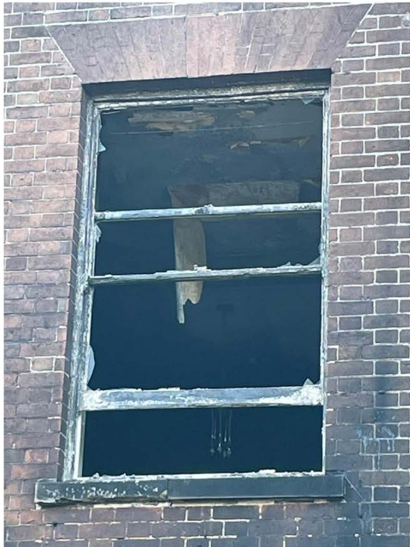
Figure 10 – Damaged timber window externally to first floor hotel room.
