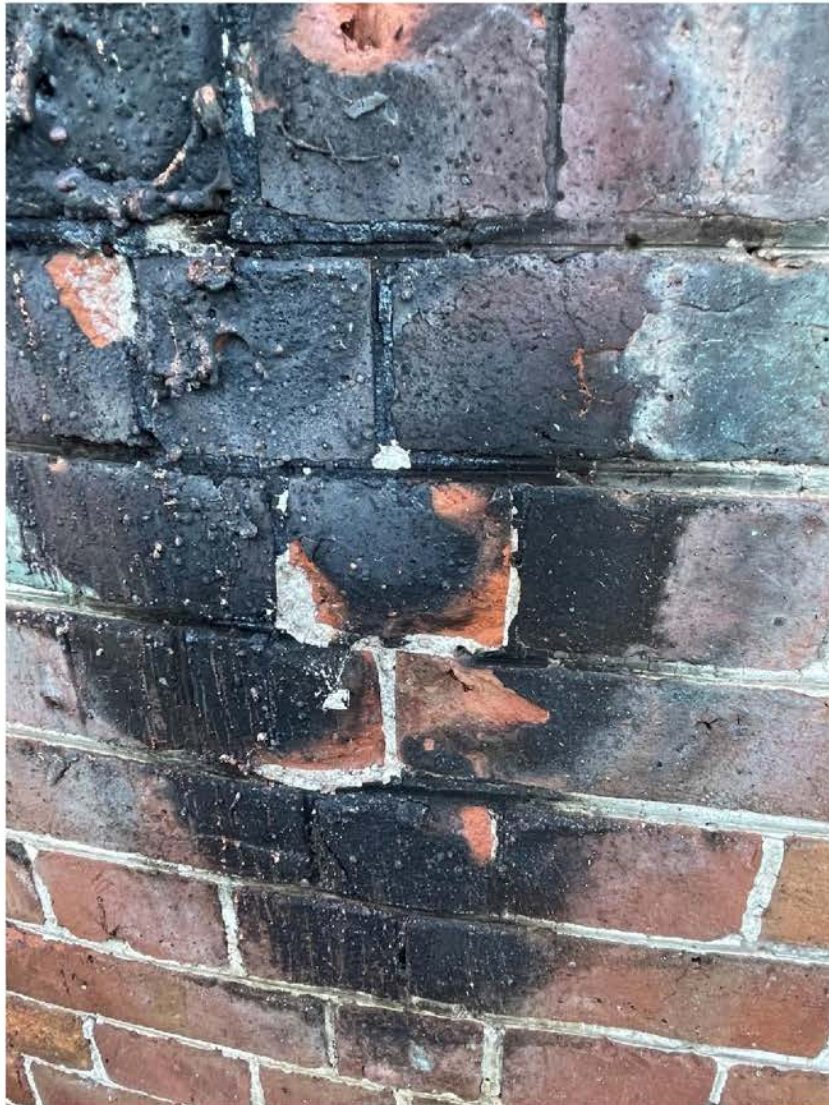
Figure 9 – Damaged brickwork following fire to rear elevation.
