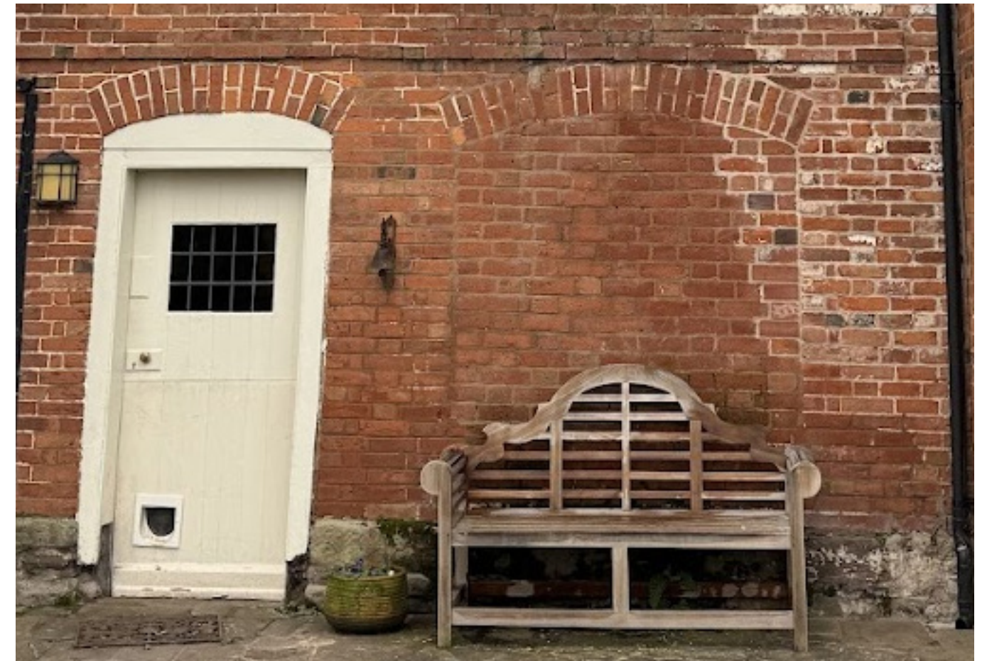
Photo showing bricked up window with its cementitious pointing.
