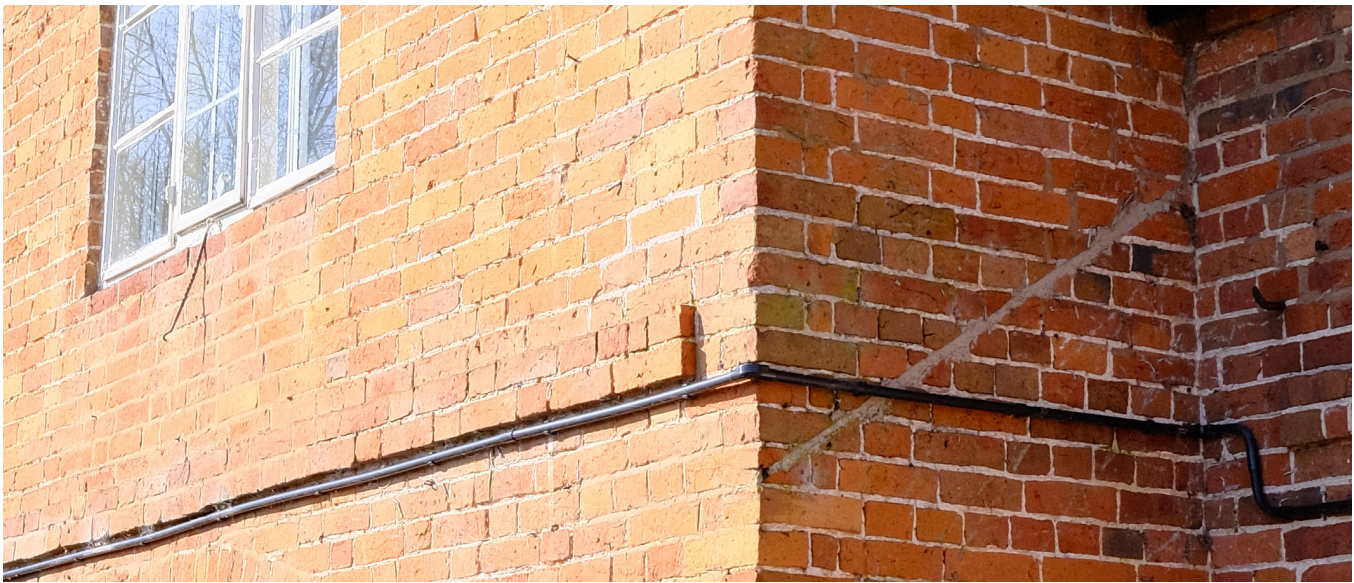
Original flashing line of leanto conservatory on return of brickwork
