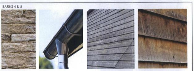
latural Barn detailing to be kept simple and agricultural. Natural lime pointed stonework, Oak timber cladding will age and soften naturally and retain a rural barn like appearance. Oak joinery left to silver with galvanised guttering and plain clay tiled roof.
