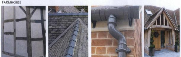
vatural Oak repaired frame walls with lime rendered panels, oak weatherboarding, traditional welsh slate root and oak joinery details will enhance he historic asset. Materials used on the Existing Farmhouse to be historic yet residential detailing. Natural quality slate roof, cast iron guttering, oak window and lime rendered infill panels.
