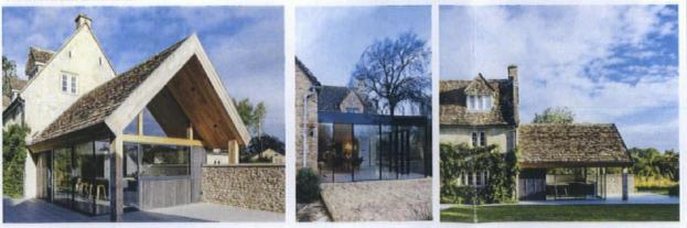
Mixed natural materials, subservient wall treatment and glazed links visually lower the structure into the landscape and reduce visual mass.
