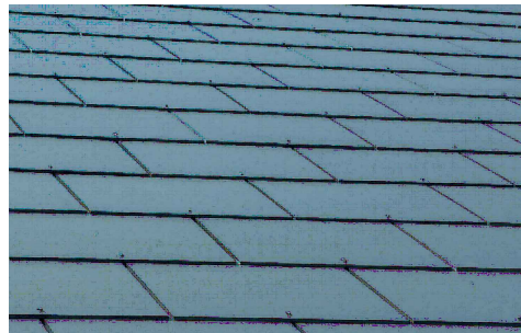
'Cembrit' Jutland fibre cement roof slate colour blue/black - all plots
