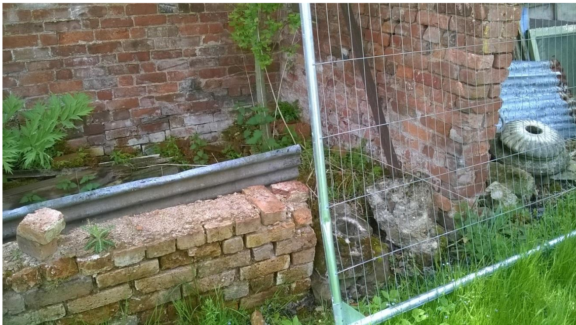
Figure 6: Plinth wall with considerable lean – to be demolished
