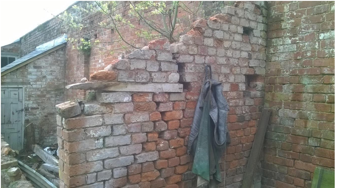
Figure 8: Other side of Cross wall showing no tie-in
