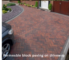
Permeable block paving on driveway
