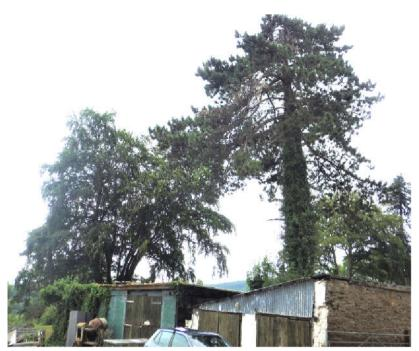
The building to the left is separated from the pine tree by a strip of rough, sloping ground with a trench dropping down to the rear of the building. It is clear that the roots system of the trees will have been tightly constrained by these structures and, depending on the relative ages of the tree and the buildings, may have resulted in significant root disruption.
