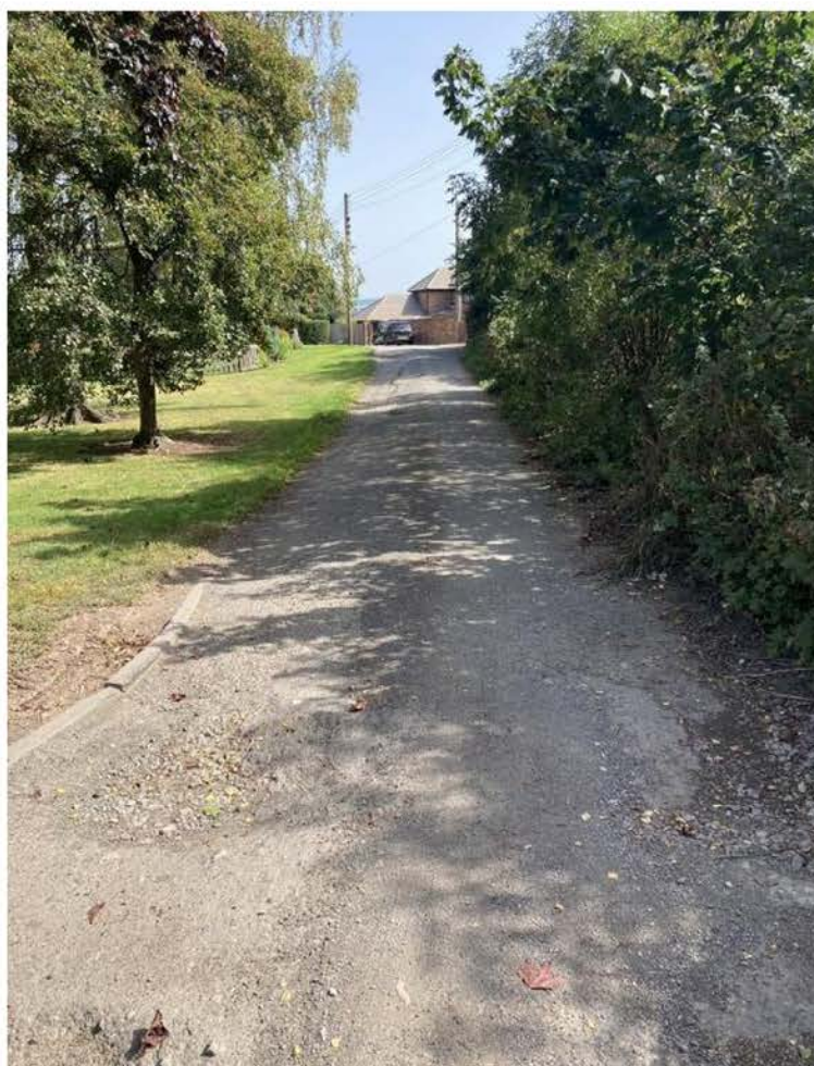
Photo 4.1 Existing Conditions along Proposed Pedestrian and Cycle Link
