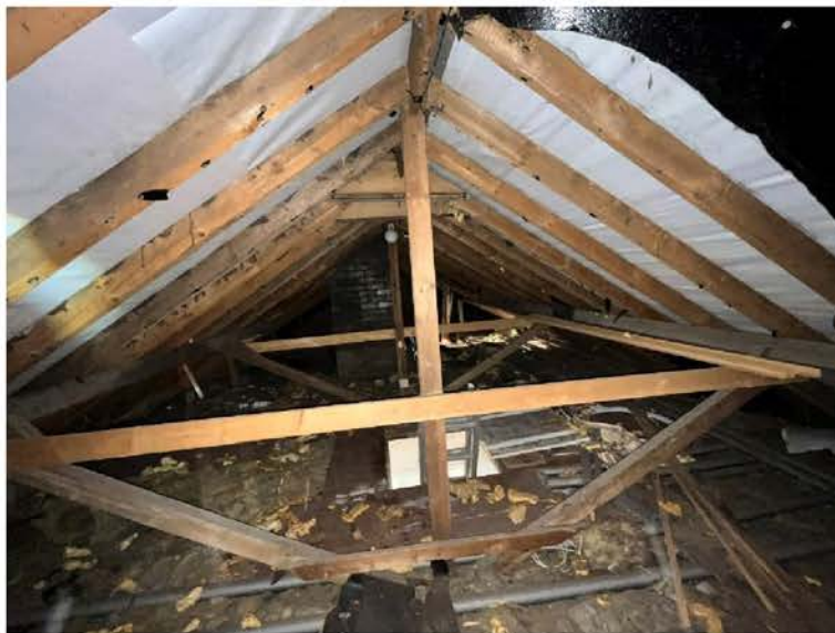
Plate 10. General view of interior roof void, note the use of breathable roofing membrane.
