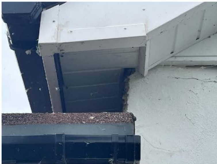
Plate 4. Unfinished soffit boards on south-eastern corner.
