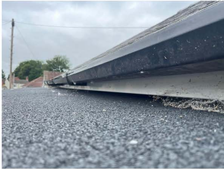
Plate 5. Gap between fascia and flat roof on southern aspect, soffits are unfinished in these locations.
