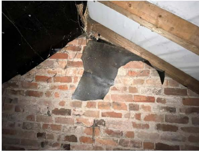
Plate 11. Remnants of bituminous felt attached to the underside of rafters.
