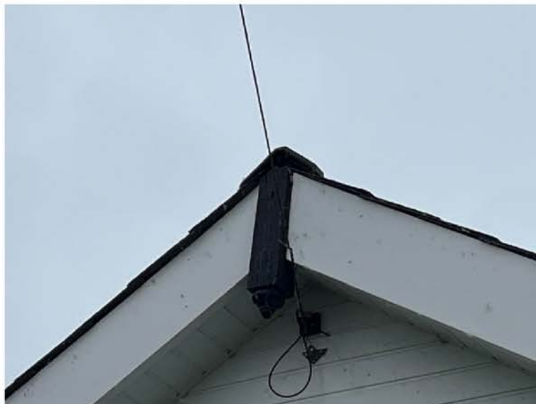
Plate 8. Un-pointed ridge tiles on gable ends provide access to beneath ridge tiles.
