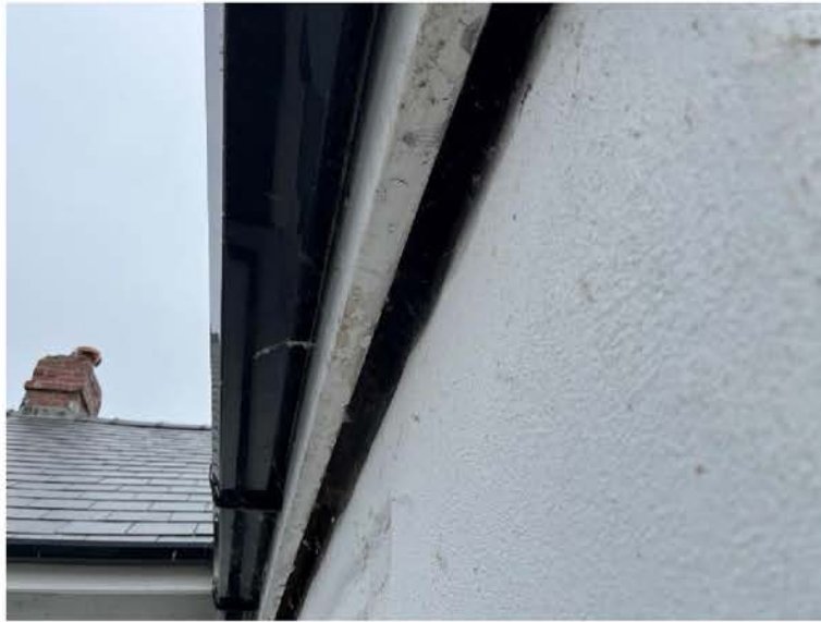
Plate 3. Crevice behind fascia board on southern outcrop extension.
