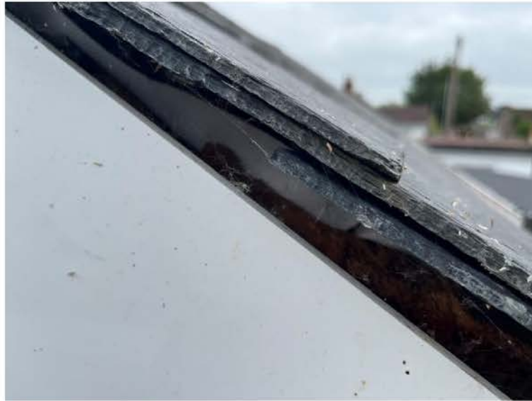
Plate 7. Un-pointed gable verges provide access to beneath slates.
