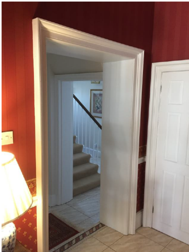
Existing doorway from the Dining Hall to the east service corridor. A new panelled door is to be inserted in to the existing doorcase.
