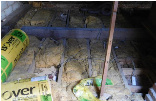
View of beam supporting ceiling joists at attic level.
