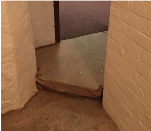
View of raised screeded floor in the Cellar. Flagstones continue under the screed and are separated by a plastic damp proof membrane.
