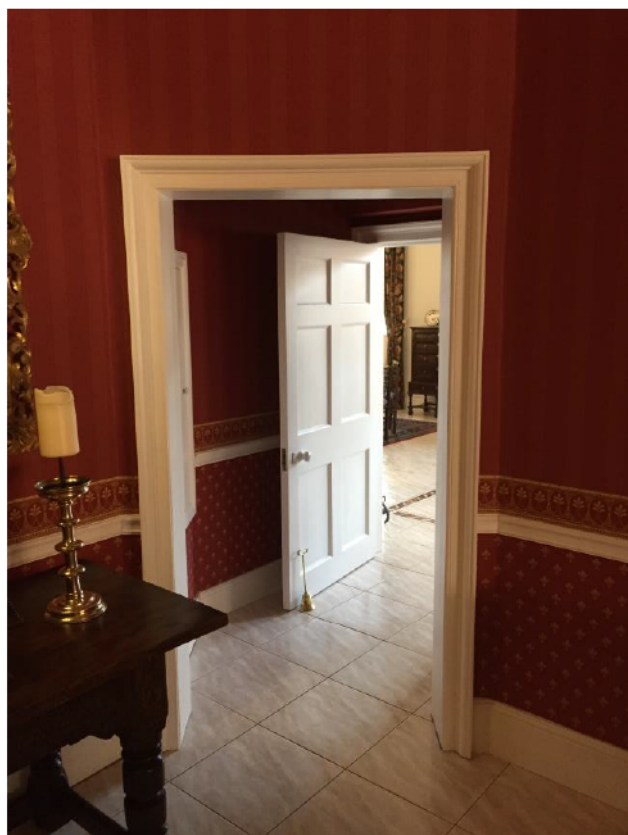
Existing doorway from the Dining Hall to the kitchen. A new panelled door is to be inserted in to the existing doorcase.
