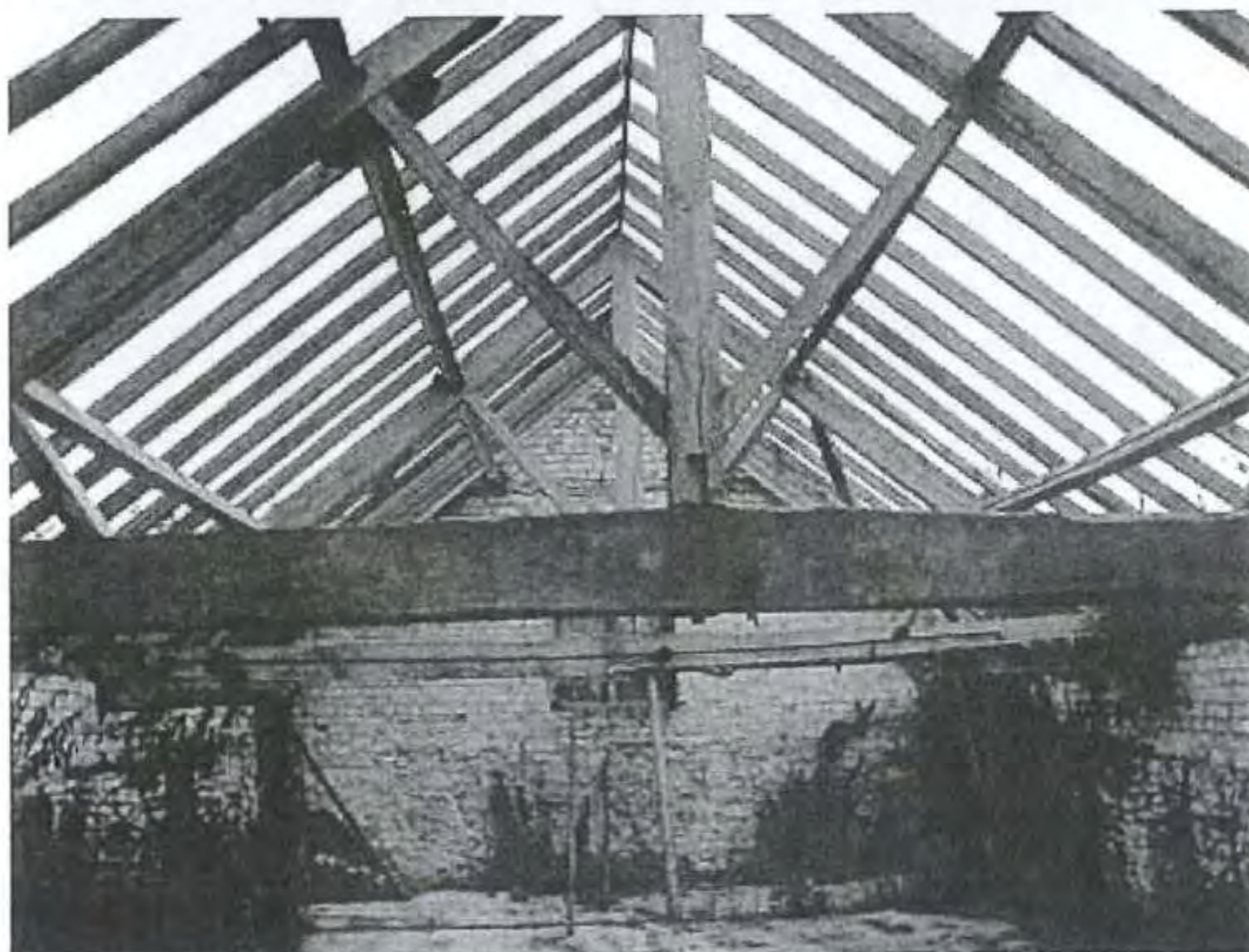
Fig 8. Inside Lower Room describing the rafters. The eaves are almost level with surrounding ground
