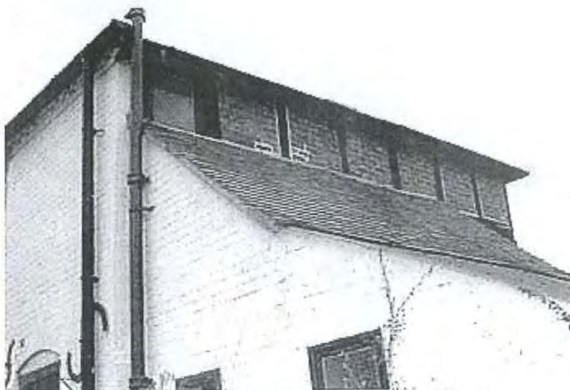
Fig 12. Describing the distance between ridge of lean too and eaves of house.
