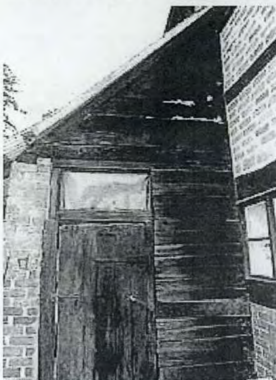
Fig 10. Close up view describing the weather lap boarding.
