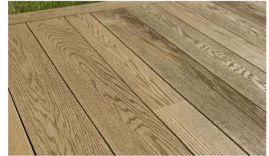
FIG 38 – NON-SLIP COMPOSITE BOARDS USED FOR DECKED AREAS
