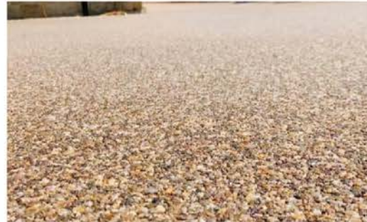
FIG 36 – EXAMPLE OF RESIN-BONDED GRAVEL PROVIDING A LEVEL, SMOOTH, SURFACE FOR PATHS AROUND THE CARE HOME
