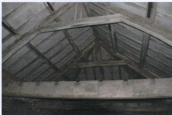
Image 4: inside view of the stables showing hipped roof and trusses with ceiling boards between rafters
