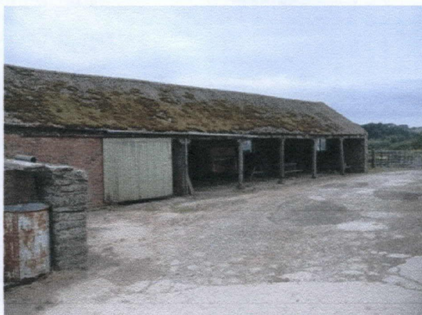
Image 5: north-east elevation of the cart shed showing open frontage and moderate condition of the roof
