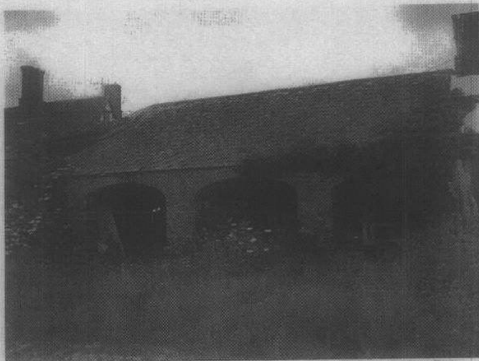
4: View of the single storey "cart shed" showing the open front and clay tiled roof
