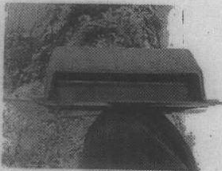
5. Plastic tile with entrance slot for bats.
