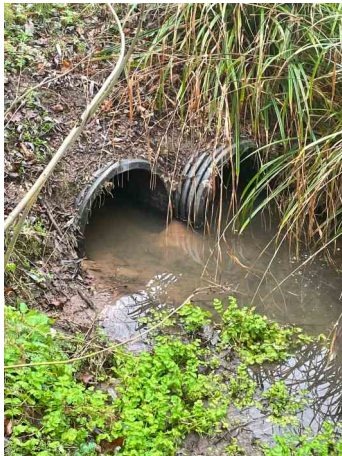
OUTFALL PIPES HOLDING 50% WATER LEVEL DUE TO DITCH WATER LEVEL
