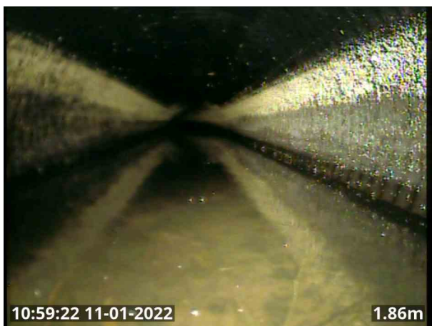
2022_01_11-10_59_23_064.jpg, 00:00:45, 1.90 m Water level, 25% of the vertical dimension
