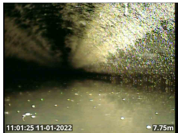
2022_01_11-11_01_26_009.jpg, 00:02:42, 7.80 m Water level, 60% of the vertical dimension
