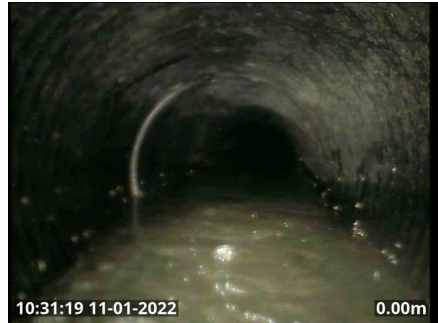
2022_01_11-10_31_19_194.jpg, 00:00:09, 0.00 m Water level, 25% of the vertical dimension
