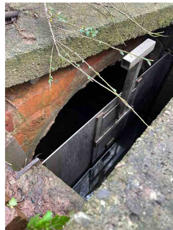
GATE VALVE FOR POND
