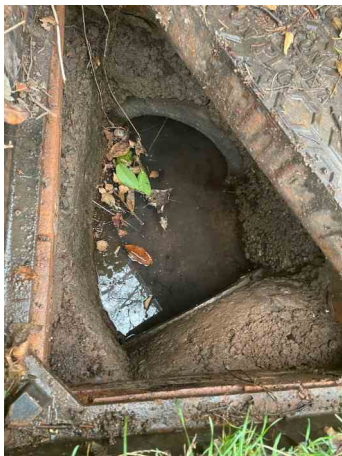
SW3, 0.98M HOLDING HIGH WATER LEVEL AND HEAVILY SILTED
