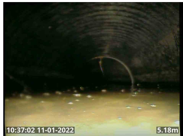
2022_01_11-10_37_02_677.jpg, 00:03:51, 5.20 m Settled deposits, fine, 30% cross-sectional area loss
