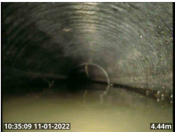
2022_01_11-10_35_09_735.jpg, 00:02:03, 4.40 m Water level, 50% of the vertical dimension
