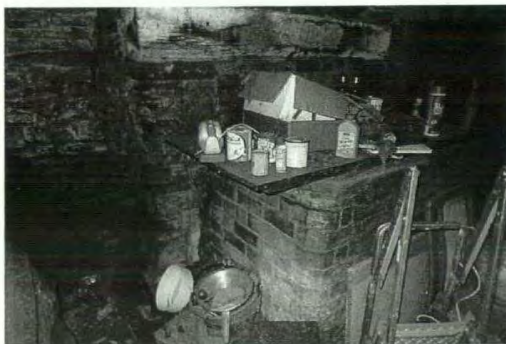
10. The 19 th century water boiler in front of the fireplace would be removed to allow the fireplace to be opened up
