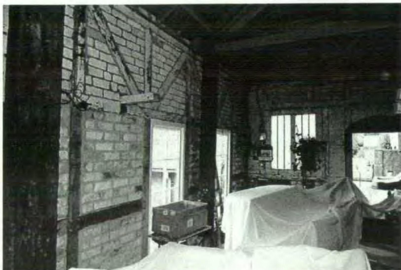
14. The external walls to the front and to the garden are only single skin brickwork and need to be thermally insulated and lined for the room to be viable for more than occasional summer use..
