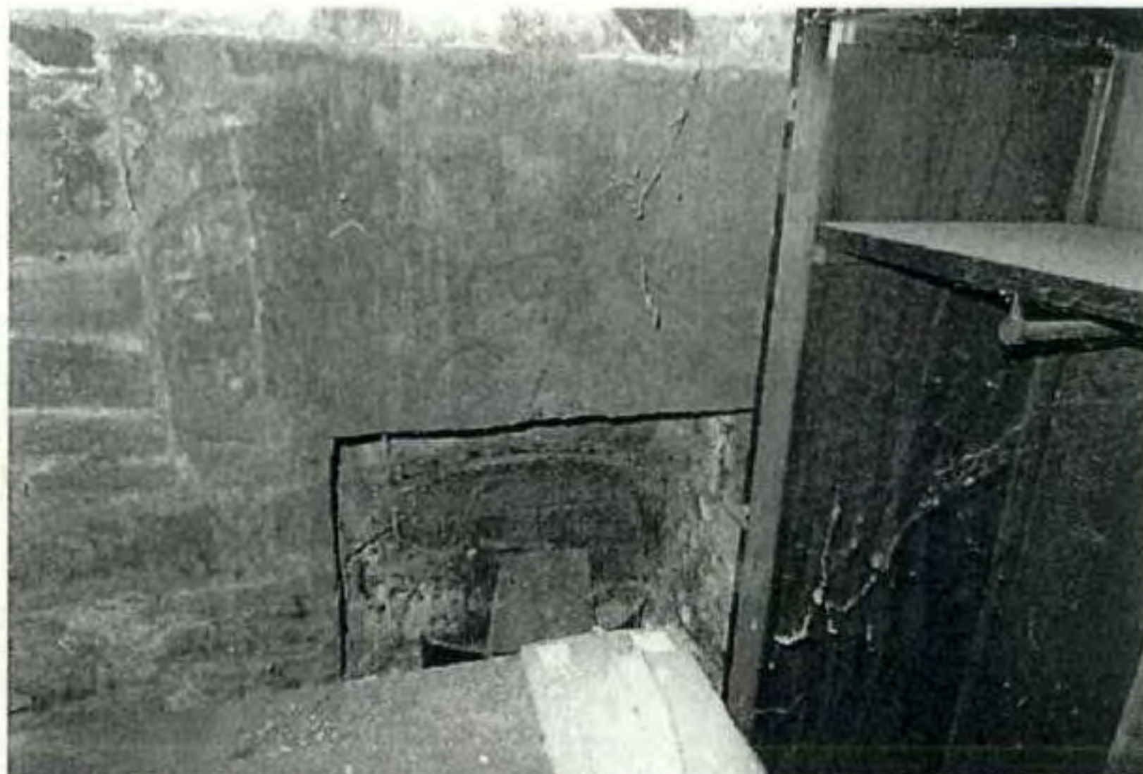
11. There is a bread oven under the stone lintol at the side of the fireplace. It appears to be intact.
