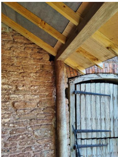
Missing wall plate and temporary repairs
