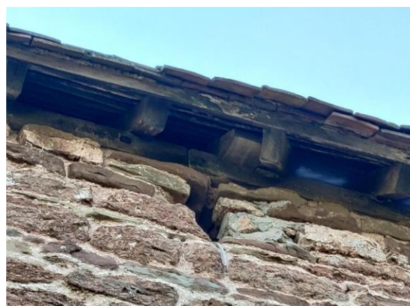
Lack of guttering causing erosion to wall and ground around the building
