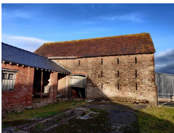
Lack of guttering causing erosion to wall and ground around the building
