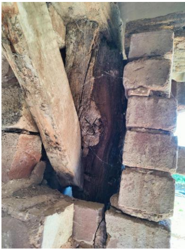
Brick infill and brick encapsulation of the original posts
