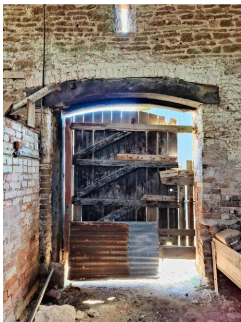
Decay in the wagon doors front and rear.
