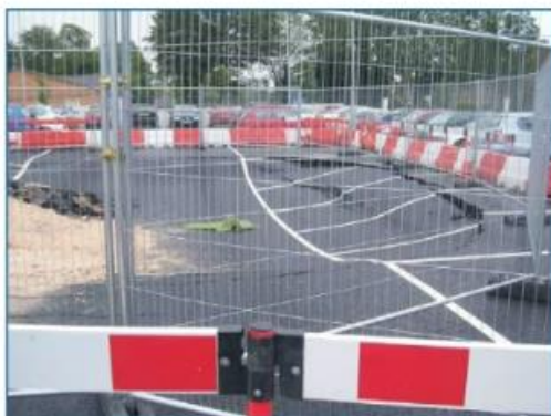
Loss of use of car park spaces due to tank collapse
