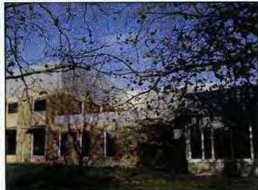
Areas of low level where trespassers access.
