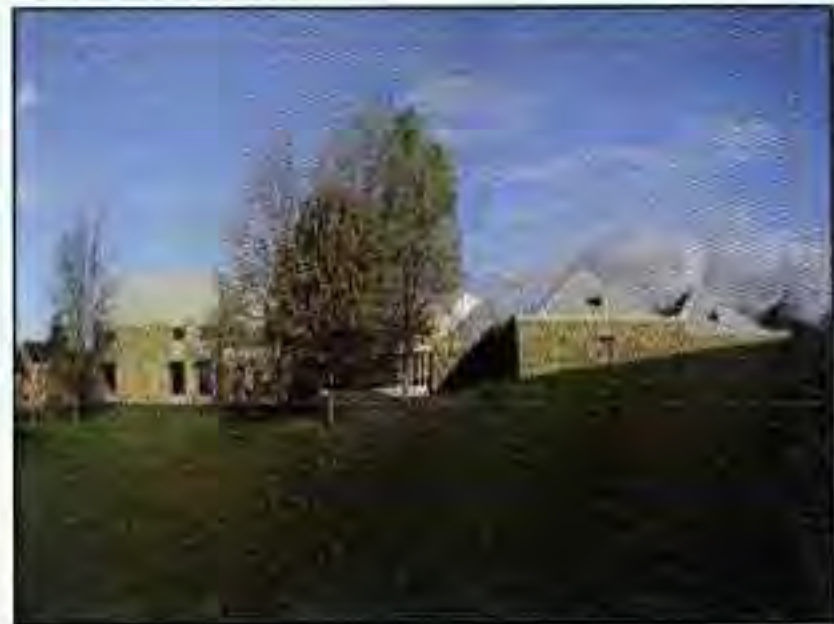
Areas of low level where trespassers access.
