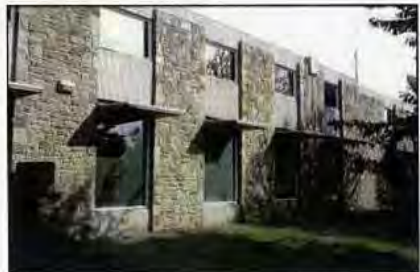
Replacement of doors and windows.
