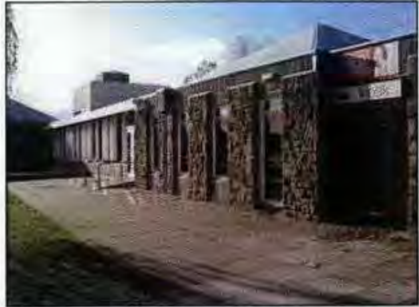
Areas of low level where trespassers access.
