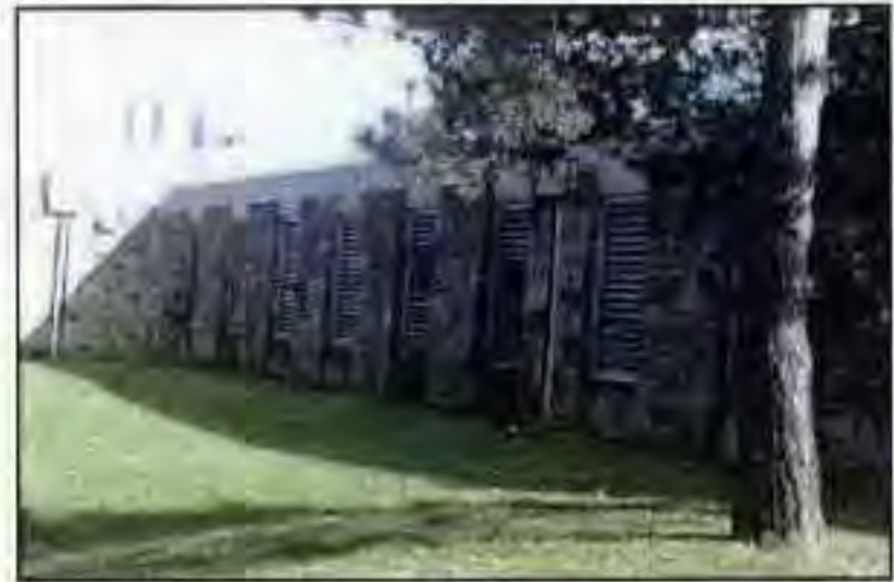
Elevation where external cladding will be installed.
