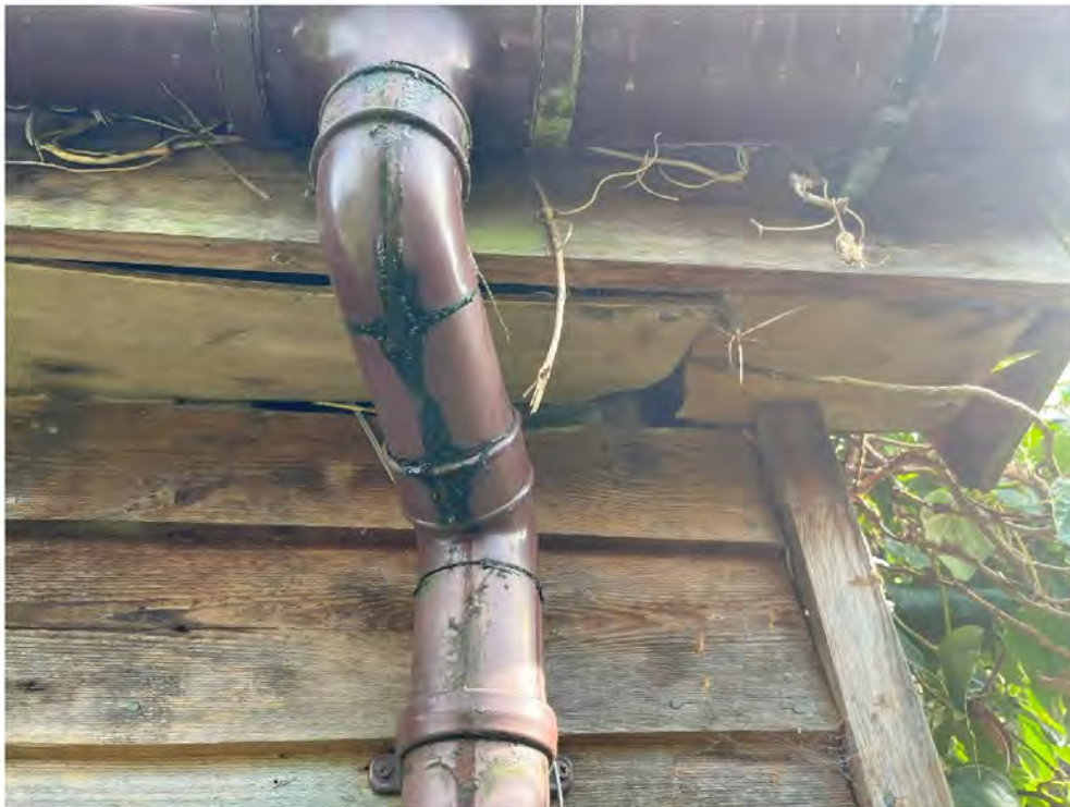
Plate 3. Damage to soffits on south-western corner of barn providing access to interior.
