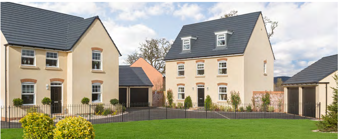
Attractive properties fronting open space at King's Wood Gate.
