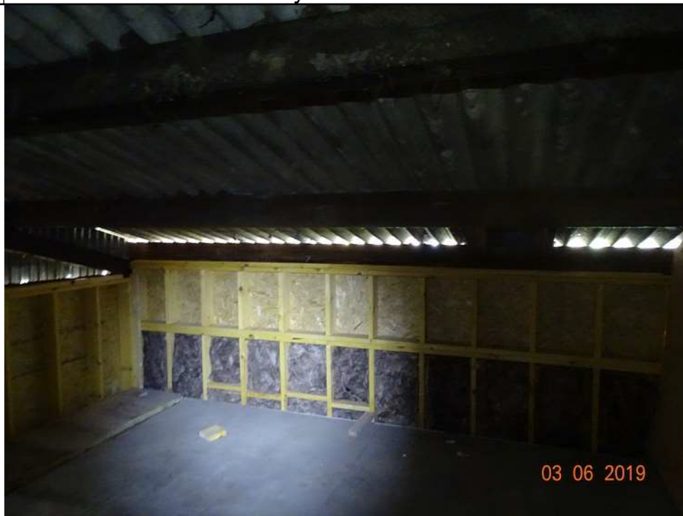
Fig 4. Describing the amount of light entering loft from eaves.
