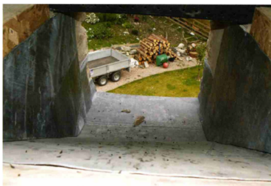
View looking down hopper to outside. Droppings visible on lead.
