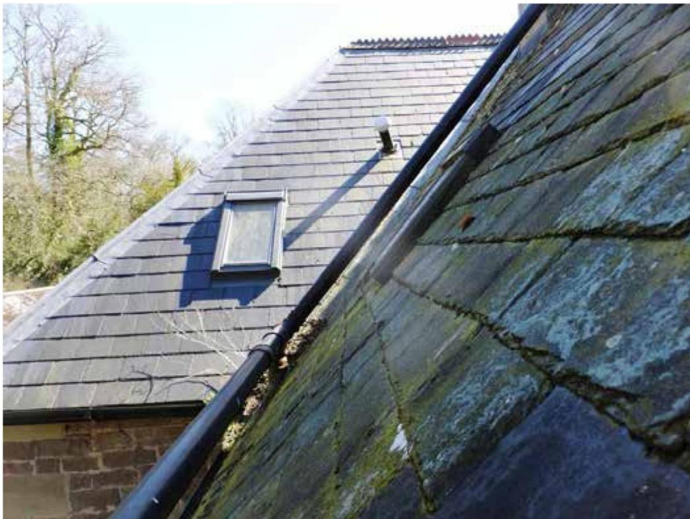
Bodenham Manor. Exterior. View of part of the Northeast elevation roof structure of Section A. Left: part of the 'recently' re-covered hipped roof. Right: part of the main Northeast elevation roof-slope.
