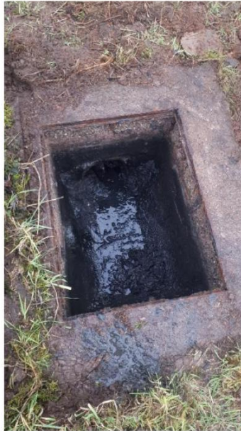
Outlet inspection chamber
