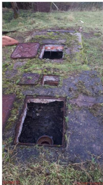
Septic tank and outlet inspection chamber.
