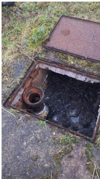
Two dip pipes in good order.
