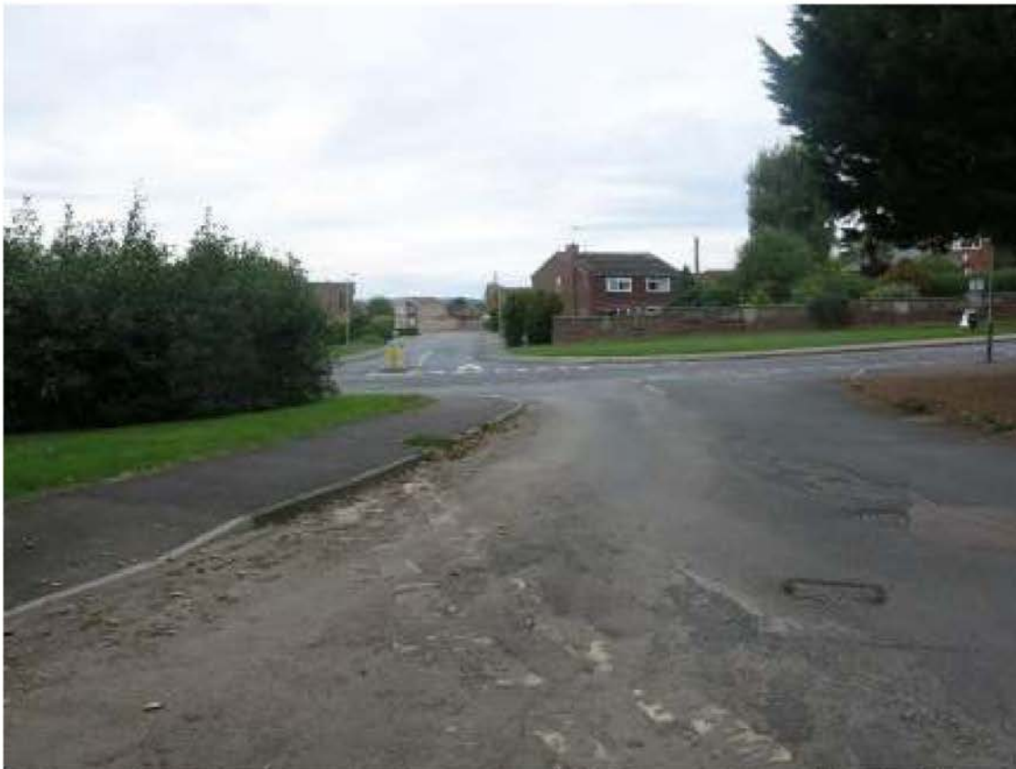
VISIBILITY LOOKING WEST AT EASTFIELD ROAD JUNCTION @ 2.4 M SETBACK
