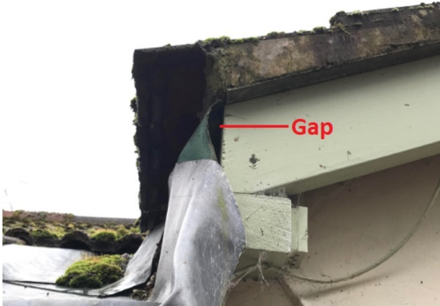
Figure 7. Gap between the lead flashing and a bargeboard on the northern gable of the cottage.
