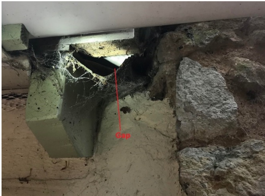
Figure 10. Gap under a fold of bitumen membrane on the north elevation of the cottage.
