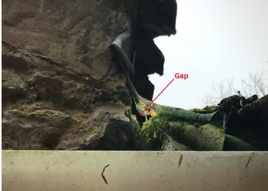
Figure 9. Gap under lead flashing on the north elevation of the cottage.
