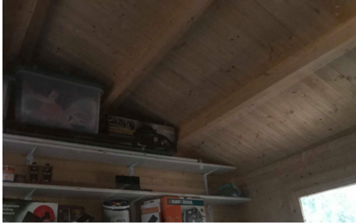
Figure 23. Internal view of the garage's ceiling and walls made with sarking boards (storage room).
