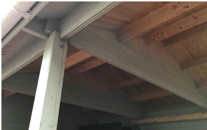
Figure 24. Internal view of the garage's ceiling and walls made with sarking boards (shelter).
