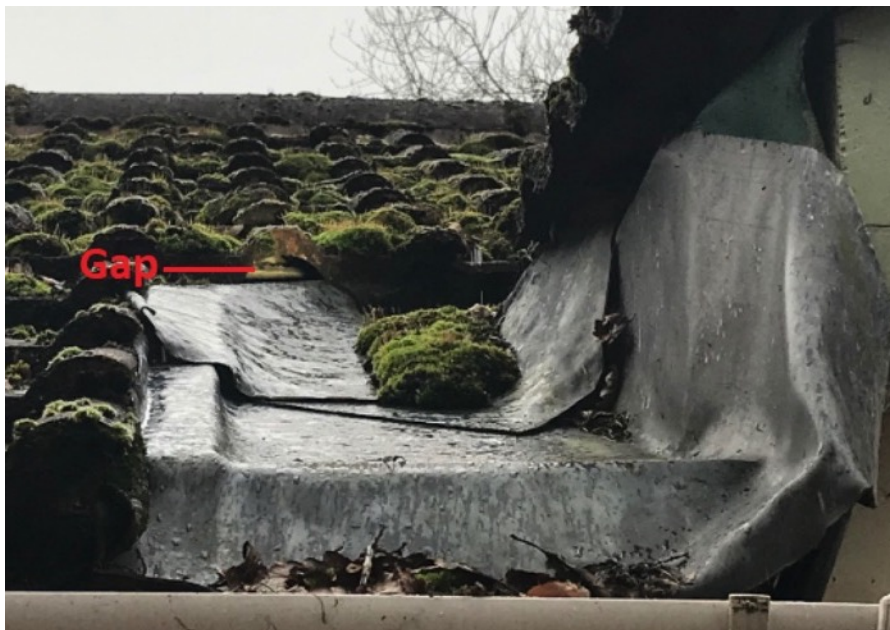
Figure 8. Gap under a roof tile on the north elevation of the cottage.
