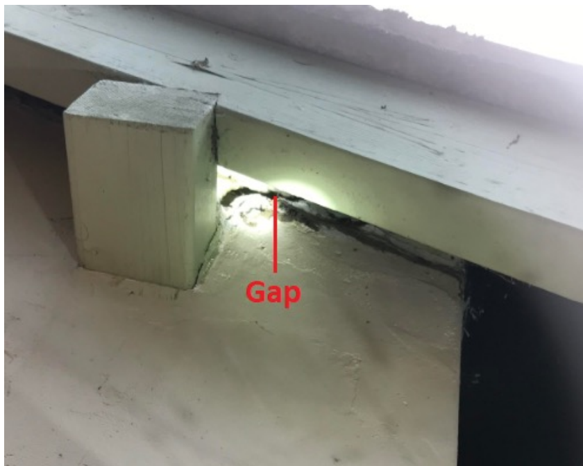
Figure 6. Gap in the masonry on the north elevation of the cottage.
