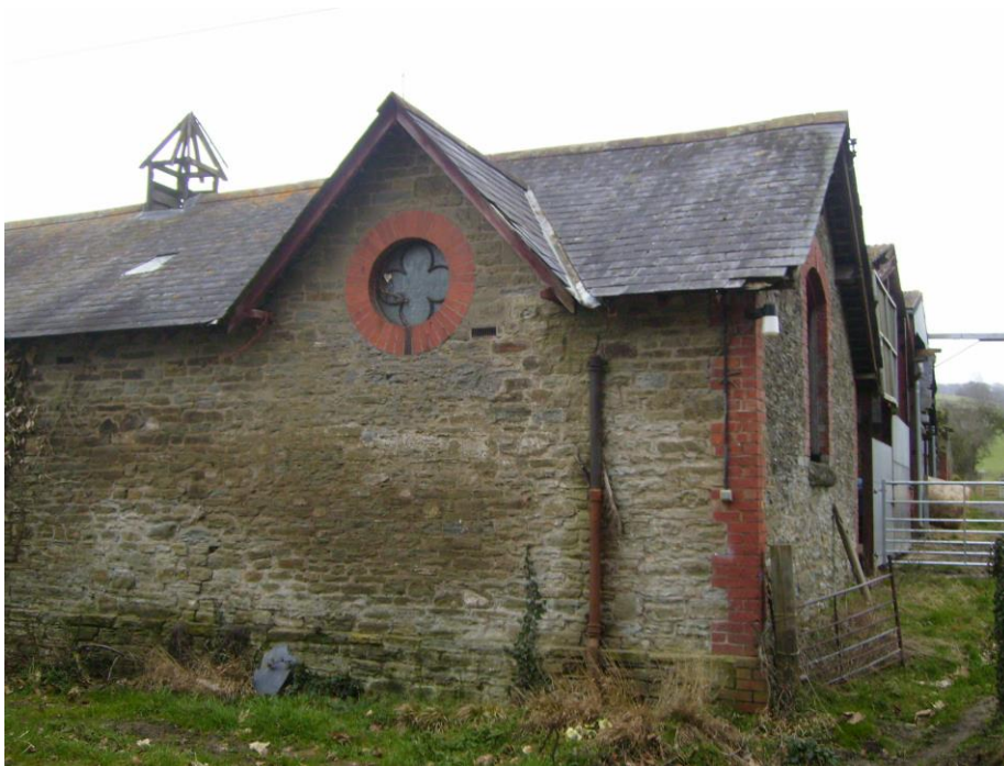
Round windows & metal frames to be retained in Barn 5.
