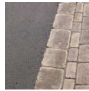
Bitmac with block paved drainage channel
