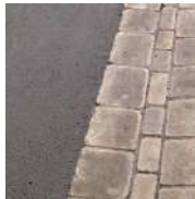
Bitmac with block paved drainage channel
