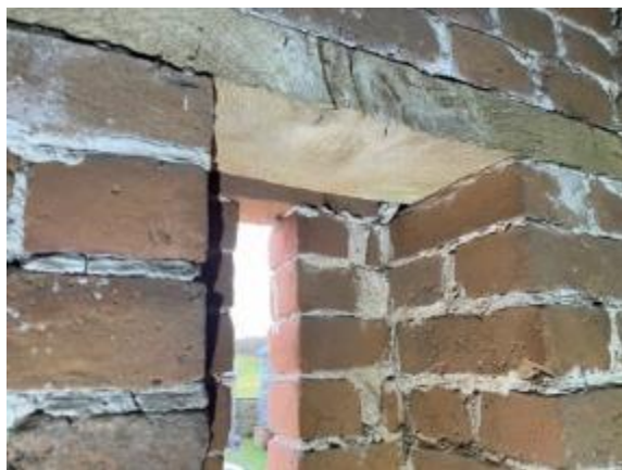
Plate 11: South barn, timber lintel within inner brick wall.
