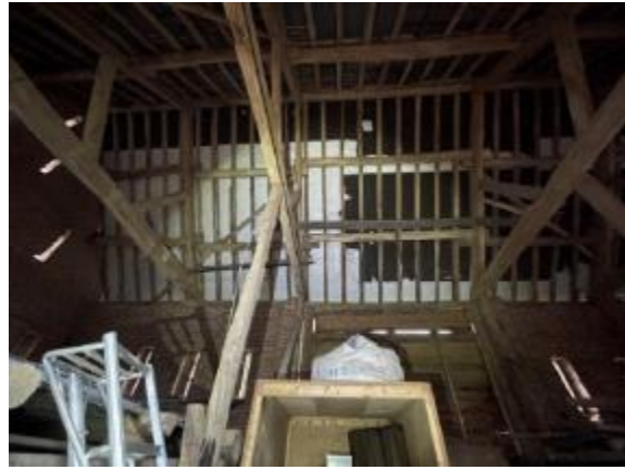
Plate 10: South barn, south roof pitch, with felt and breathable membrane lining.
