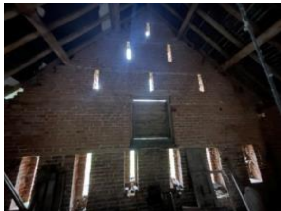
Plate 8: South barn, slitted brick vents.
