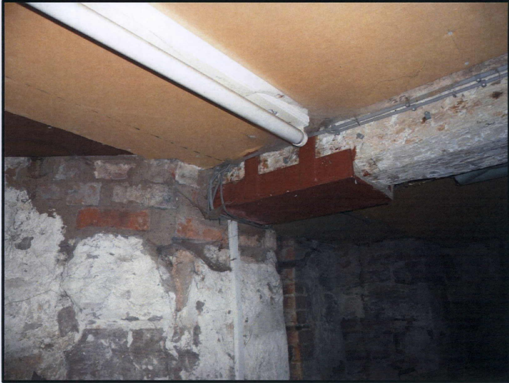
7. Steel 'shoe' to support beam end in cellar 1
