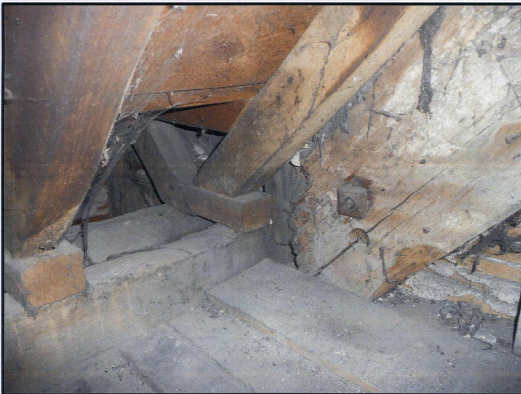
8. Historic wet rot decay to roof truss end in old tank cupboard (2 nd floor)
