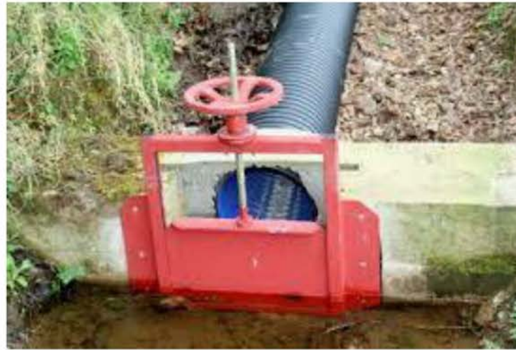
Example of the type of sluice gate control mechanism in the leat.
