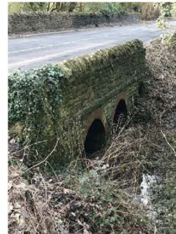
Twin culvert under A438
