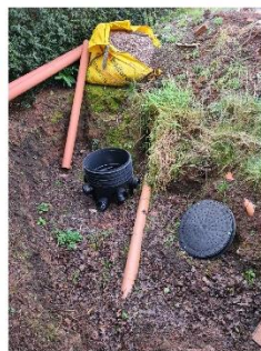
Existing outflow from STP Upstream Distribution unit Gravel Slotted outflow pipes
