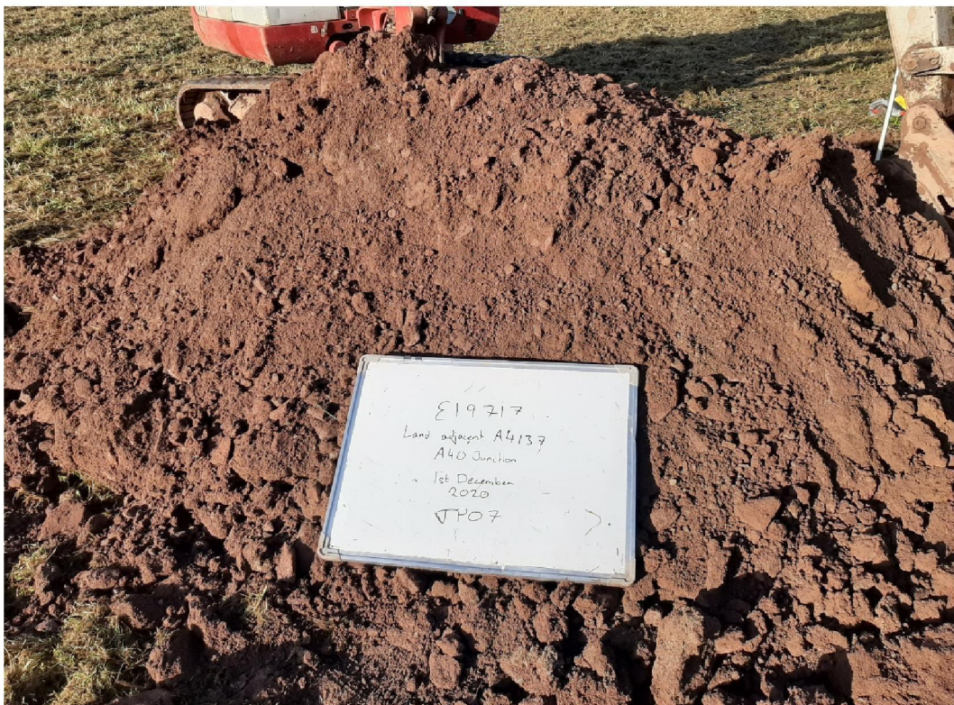
Photo 13: Trial Pit TP07
