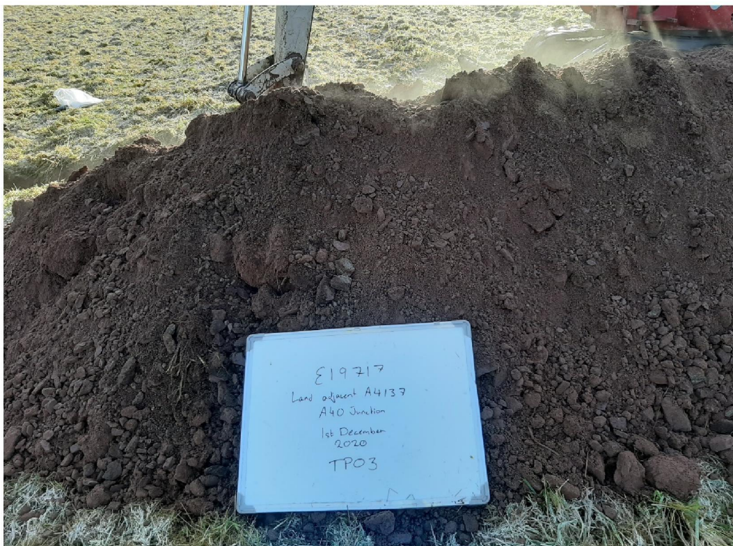
Photo 5: Trial Pit TP03
