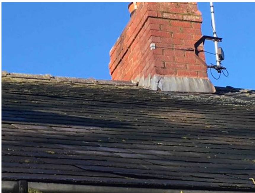
Image 16. Gap between ridge tile and chimney
