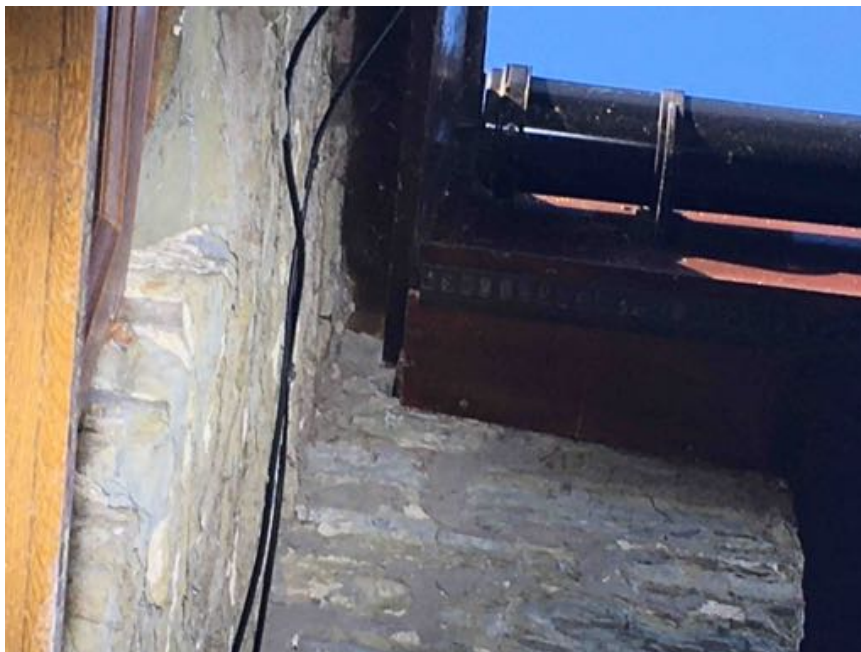
Image 14. Potential gap into soffit box on north elevation
