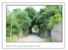
6.49 In order to facilitate the development, Cawdor Arch Road Railway Bridge feeding the main access road into the site will be reduced along with the accompanying rail embankment to facilitate full access for emergency vehicles. The lower reaches of the arch will be retained and capped off with the embankment graded up to the remnant former track bed.
