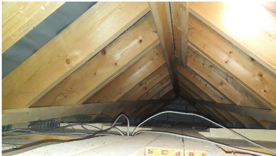
Plate 8: Target Note 2. A view of the loft space. Note the new timbers and roof-lining, and the clean floor surfaces.
