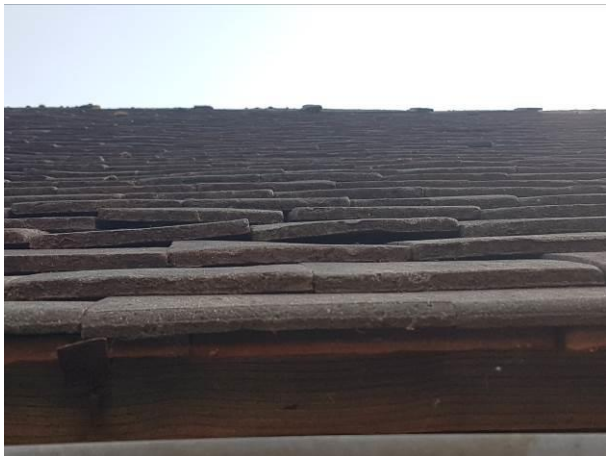
20. Gaps under raised tiles on The Wain House
