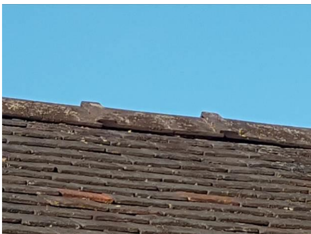
22. Gaps under ridge tiles on The Wain House
