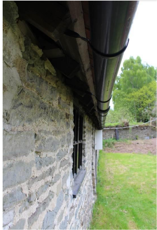
28. Gaps beneath the roof at the eaves on The Wain House
