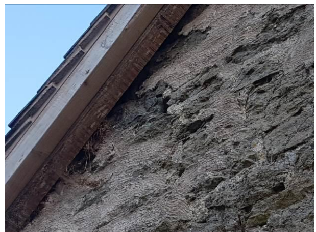
23. Gaps behind barge board on The Wain House
