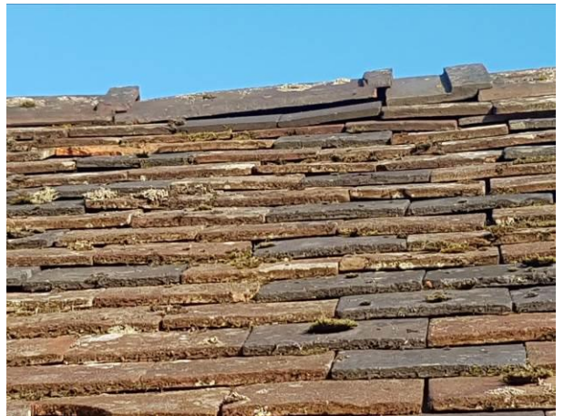
21. Gaps under raised ridge tiles on the Wain House
