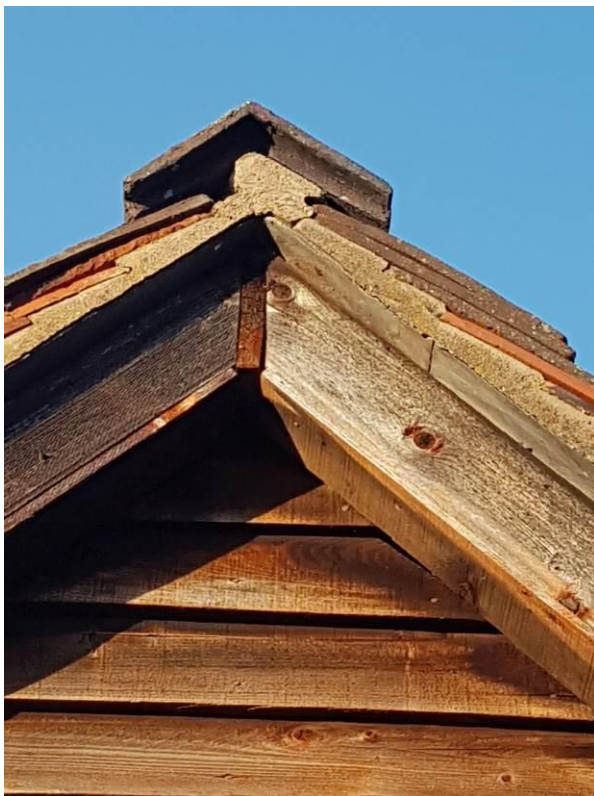
25. Gaps under ridge tile on the porch of The Wain House
