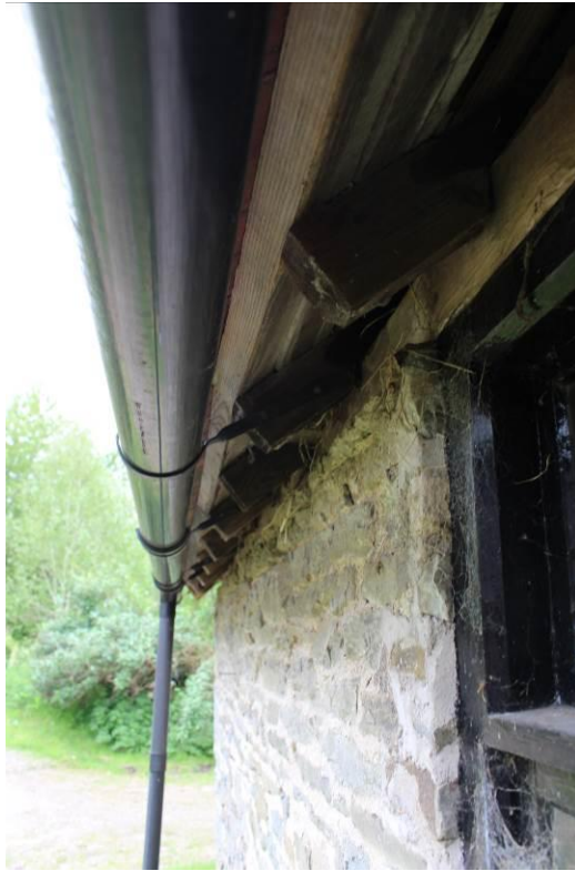
27. Gaps beneath the roof at the eaves on The Wain House
