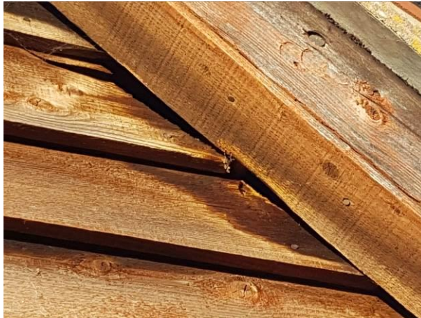
24. Gaps behind wood on the porch of The Wain House
