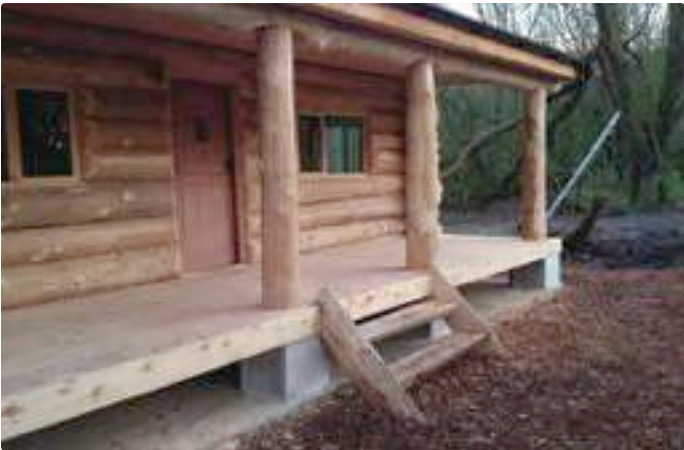
RIGHT Post and beam porch on a woodland retreat with milled Douglas Fir decking boards.
