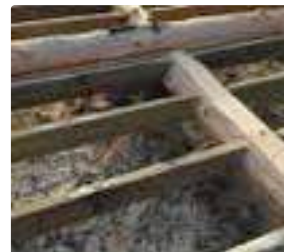
BELOW Floor joists fitted into the foundation log with a slot cut to accept the flooring.
