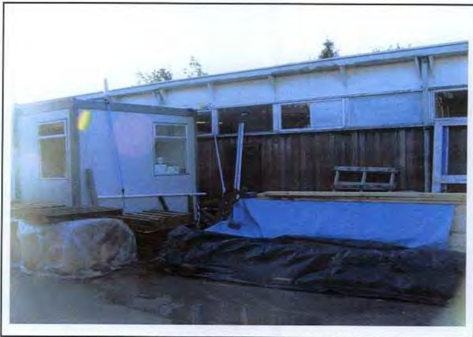
Photograph 3: Builder's Yard Area in the north of the site.
