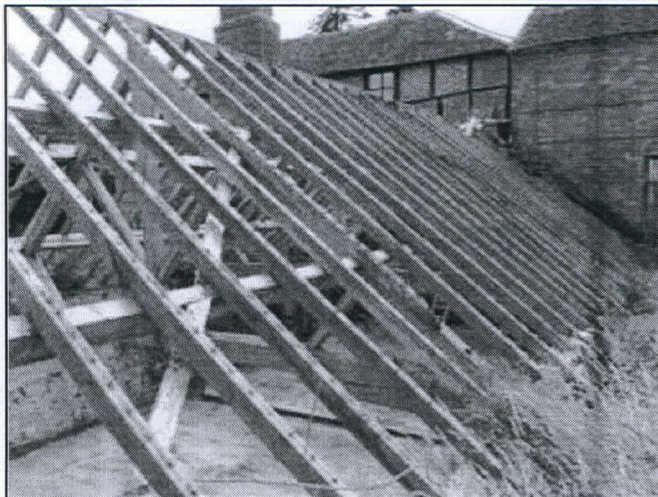
Cider storage barn: subterranean to wall plate height. Clay tiles have been removed from the weak roof timber structure and stacked nearby.
