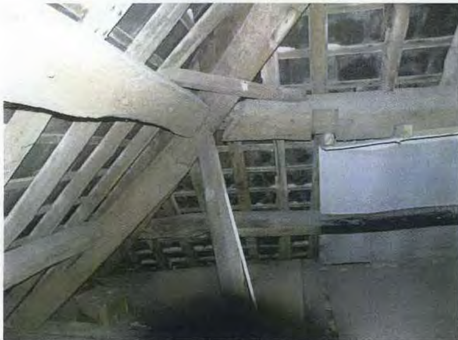
Pl.11: Detail of the hipped roof structure at the west end of the Hall Range.
