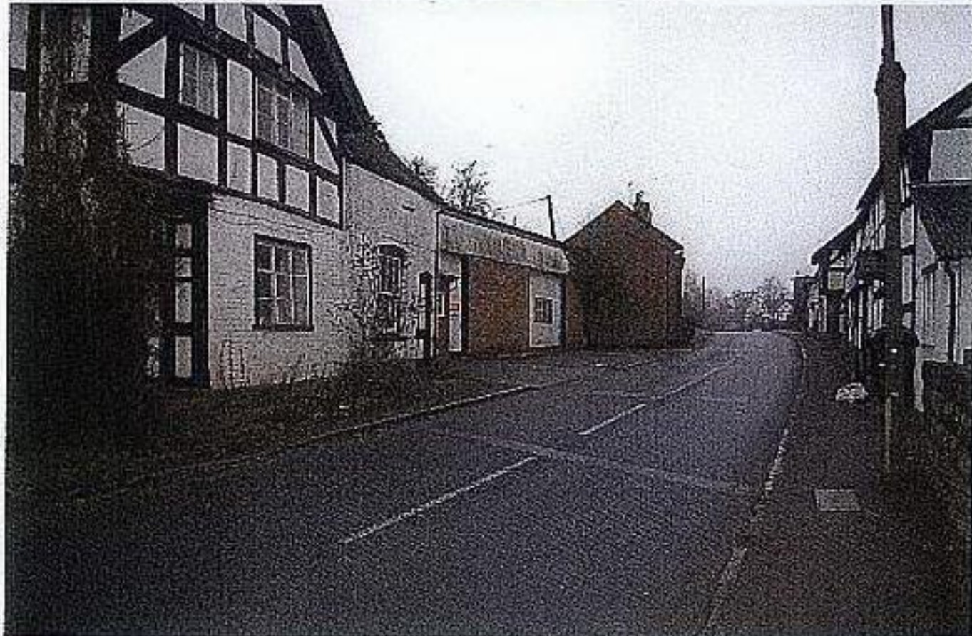
VIEW ALONG WEST STREET FACING WEST
