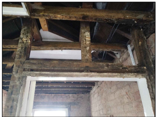
Photo 01 - Timber Partition (Timber Partition to Storeroom affected by Dry Rot to be repaired)
