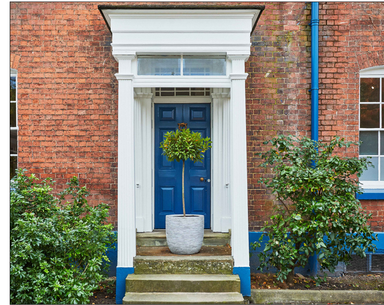
EXISTING PHOTOGRAPH OF PORCH AREA
