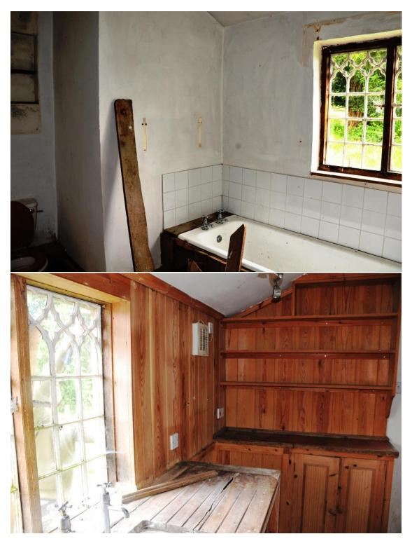
The structures have very little thermal quality resulting in internal condensation and living conditions injurious to the health of occupants. This is compounded by very awkward junctions with the original property which are both aesthetically disfiguring
