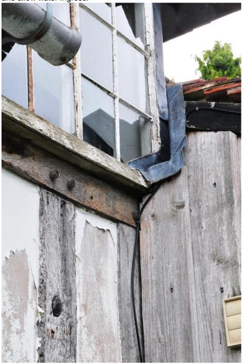
During the second half of the twentieth century the old wattle and daub panels of the cottage were replaced by modern brick and composite cement rendered units which are now breaking down and require replacement.
