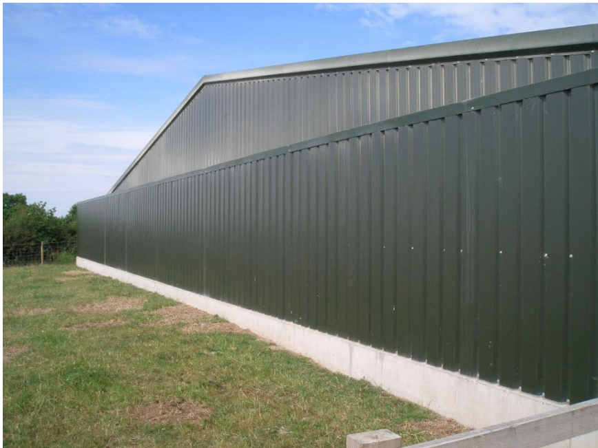
FIGURE 3: ACOUSTIC BAFFLE AT GABLE END FANS
