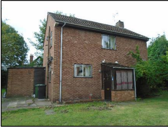
Plate 1: Showing a view of the front of the house. Photograph looking south-west.
