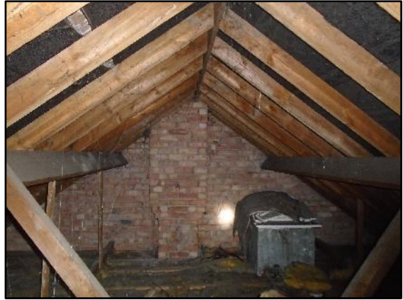
Plate 2: Showing a typical view within the roof void of the house.
