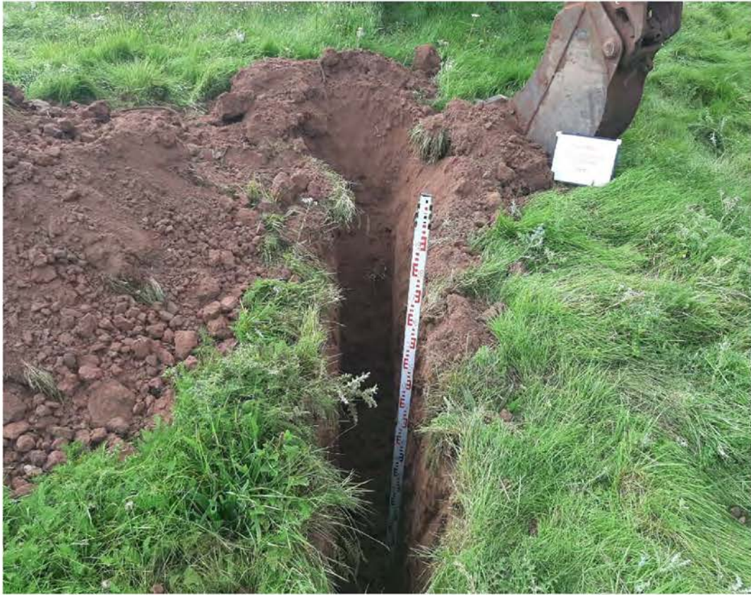
Photo 3: Soakaway Pit SA01
