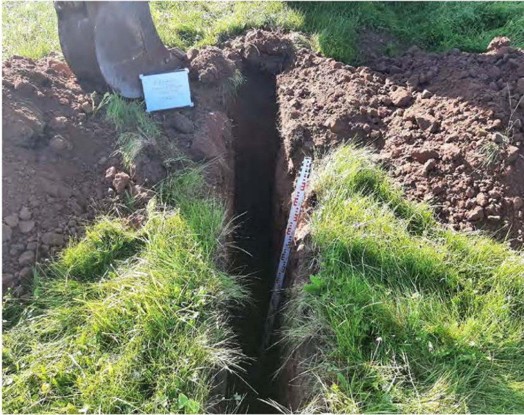
Photo 7: Soakaway Pit SA03
