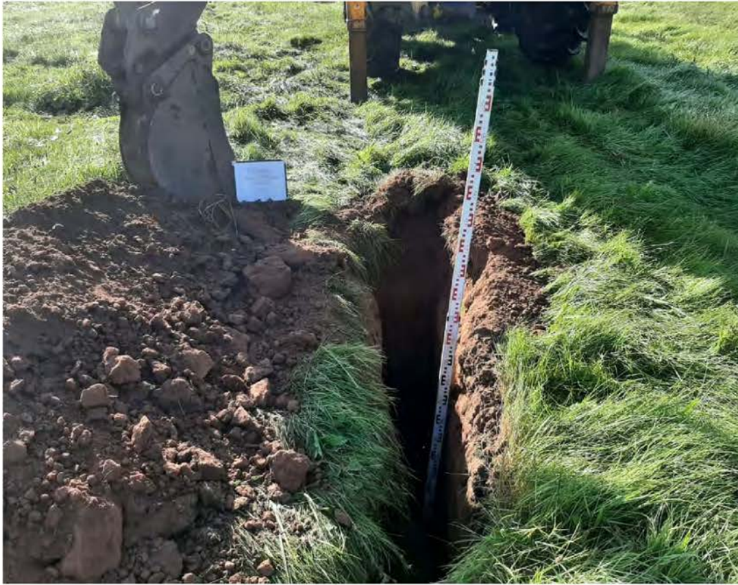
Photo 5: Soakaway Pit SA02
