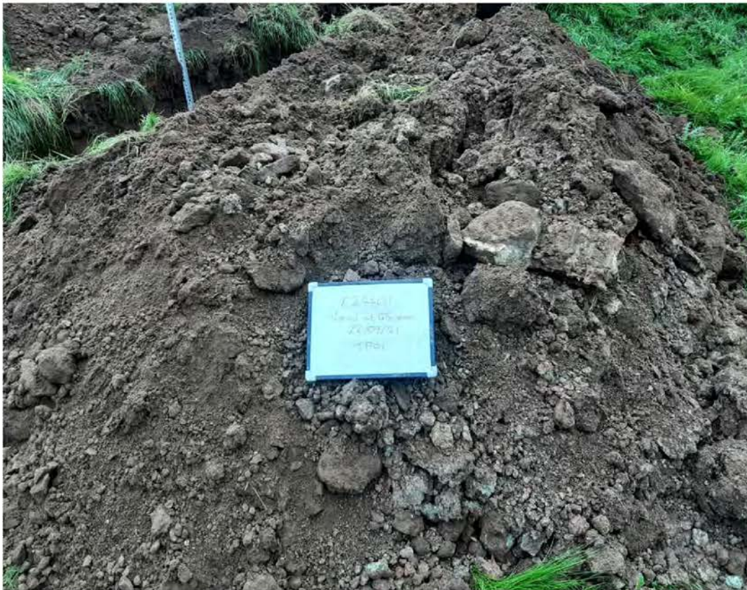
Photo 2: Trial Pit TP01 Spoil
