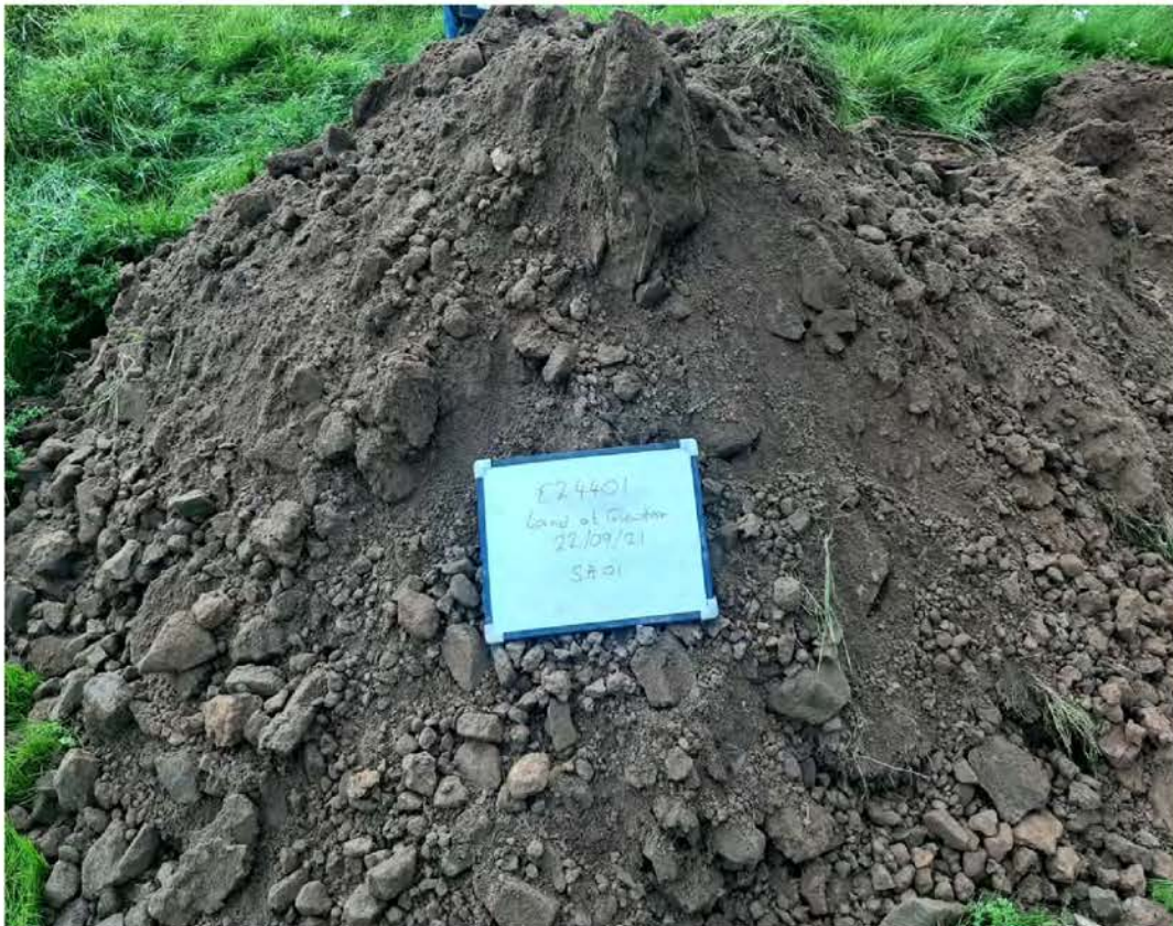
Photo 4: Soakaway Pit SA01 Spoil
